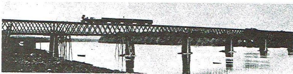
Supply train shown crossing the truss bridge in 1864. This bridge was the last one that the Federals built at Bridgeport before the end of the war. The Confederates destroyed the bridge three times during the war.
