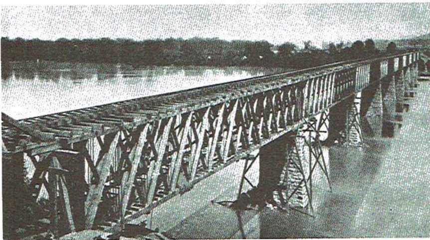
A view of the truss bridge after its completion in 1864. Notice the wagon-way below the railroad tracks on the bridge.
