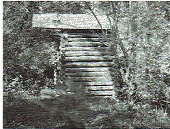
This spring house, now standing behind the Major Doran home, was used in refrigerating foods. The walls of this house were possibly built as early as 1816 or earlier. Notice the spring running from under the right side of this house.
