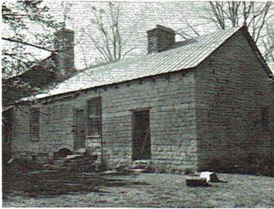
The Major Doran home, built of hand-hewn limestone, was built about 1816. The walls are 16 inches thick. Notice the portholes in the rear of the house. Major Doran was the first settler in Doran Cove, thus the cove was named in his honor.
