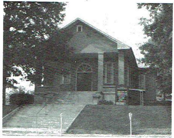
The United Methodist Church was completed in 1925.
