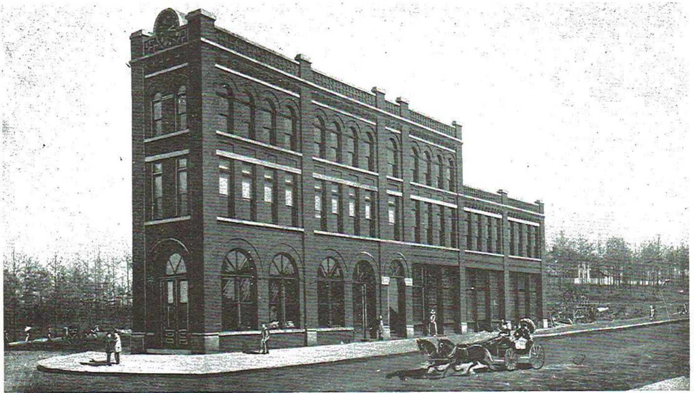
The Whitcher Block was built in 1890 by O. W. Whitcher of Boston. This building was built of pressed brick and trimmed in stone; it contained a full basement, store frontage on the first floor, offices on the second, and rooms for the Ala-Ga-Tenn Club on the third. The building was torn down in 1960.
